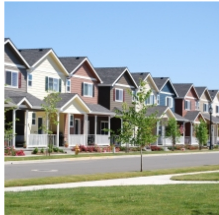
Row Houses at Twin Creeks TOD
