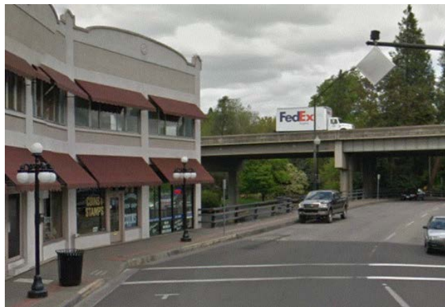
Medford I-5 Viaduct
