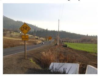
**Shoulder Bikeway:** A shoulder bikeway is a paved shoulder that provides a suitable area for bicycling, reducing conflicts with faster moving motor vehicle traffic. Most bicycle travel on the rural state highway system, and on many county roads, is accommodated on shoulder bikeways.
