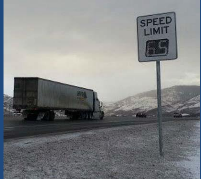
I-5: Variable Speed Limit Signs
