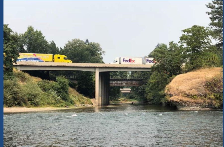
I-5 Evans Creek Bridge (Rogue River)
