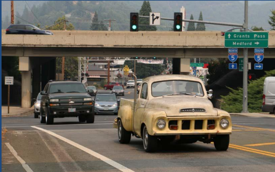
I-5 Bridge over Depot Street (Rogue River)
