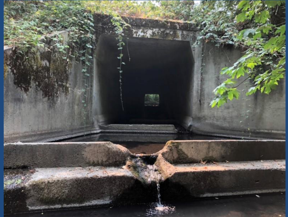
I-5: Galls Creek Culvert
