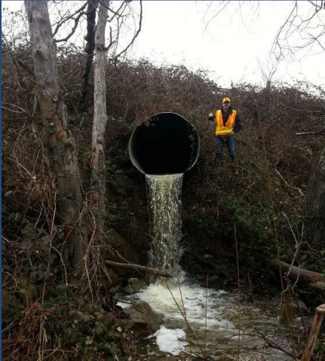
I-5: Ashland to Gold Hill Culverts
