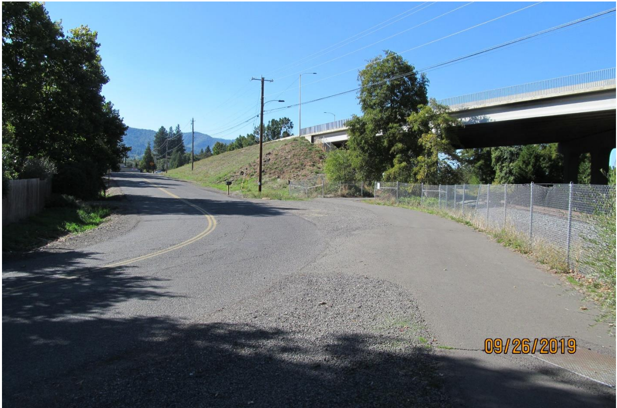
North End of Project. Note Ashland Central Bike Path on Right
